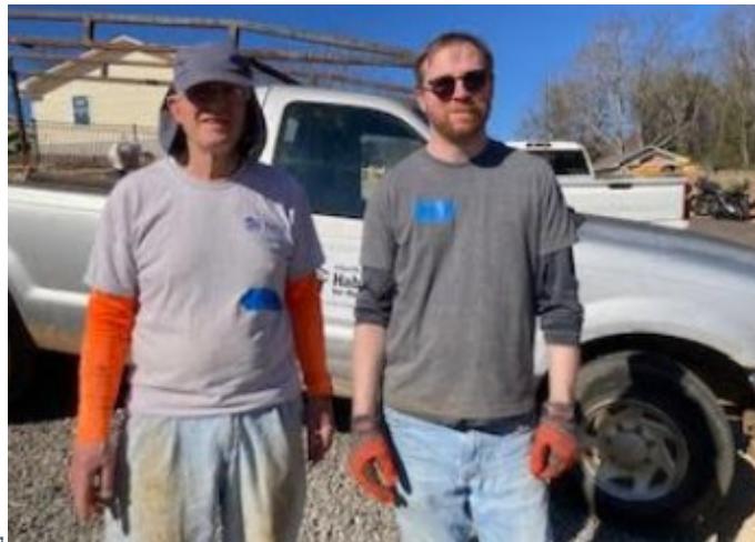
Ken Murchison and Andrew Daugherty at the Habitat site on Feb. 28. Ken, Andrew and Derron Daugherty each helped with the house building progress twice in February.
